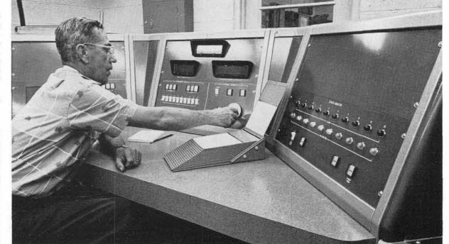
FROM THIS CONSOLE located in Bldg. 887, air conditioning and heating equipment in Bldg. 802 is monitored. System, currently being installed in Bldgs. 880 and 894, will eventually include all ma-
